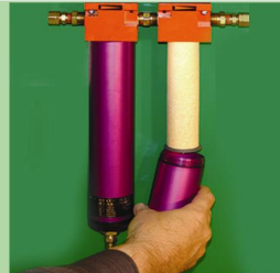
15. Remove the canister from the coalescing filter.
